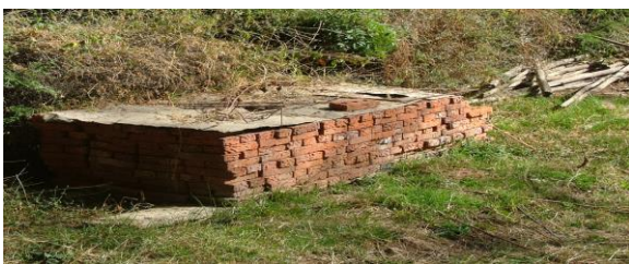
Fig 6.2 Properly stored bricks
